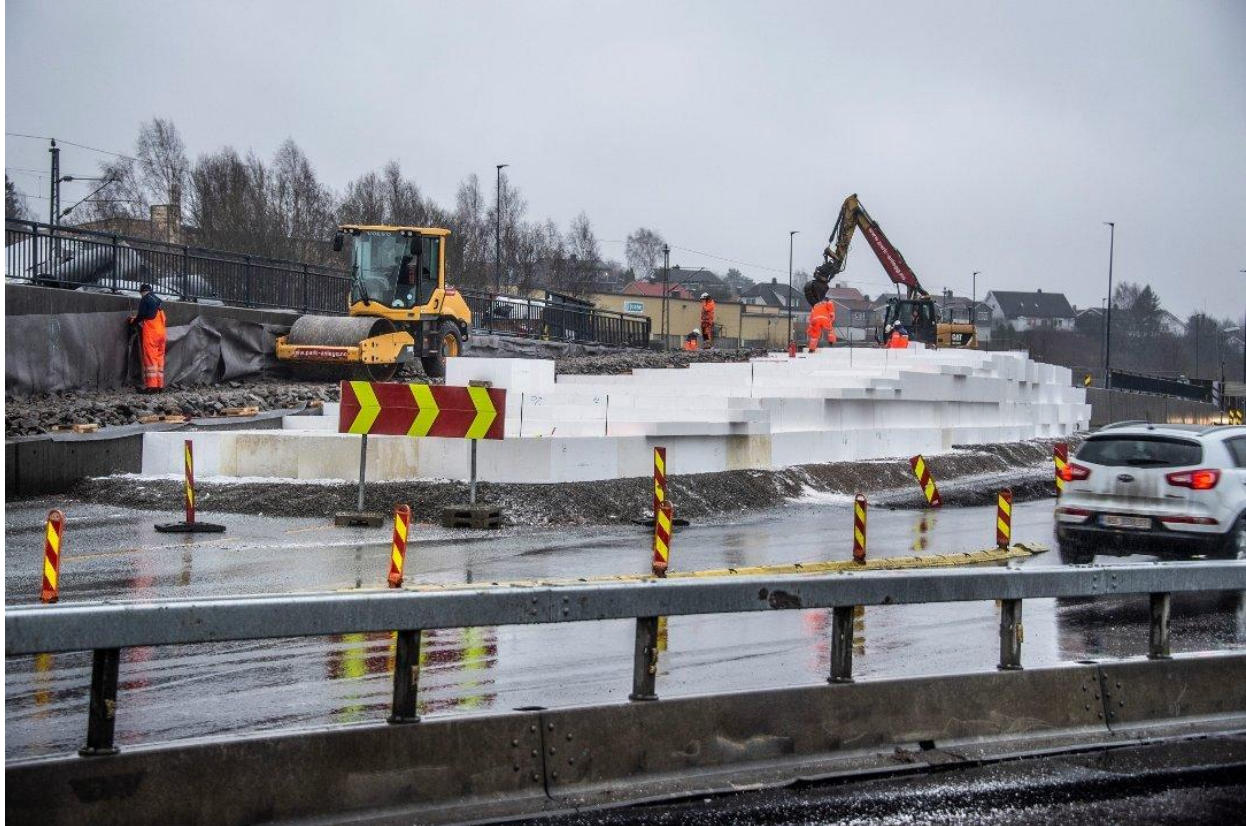
Figure 3.6: EPS as lightweight fill. Fragmented EPS litter surrounds the area. Photo: Geir A. Carlsson, Fredrikstad Blad.
